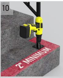
Make sure the posts are sitting a minimum of 2" from each side of the steps. Using a drill fitted with the included drill bit, drill through one of the holes on the post mount. Ensure you are drilling deep enough to accommodate the length of your fastener. For concrete, drill 3" deep, and for brick drill 6" deep.
