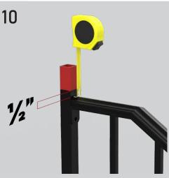
If you have not already cut the back post in step 4, do so now, making sure to leave at least 1/2" above the rail. Use the included touch-up paint to cover any bare metal that is exposed.
