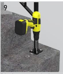
Select fasteners, appropriate for your stair material. Secure the fastener into the hole that you have just drilled. Be sure to drill one hole and secure one fastener at a time. If the post is no longer level after fastening, place the included washers under the post mounts until a level reads plumb.
