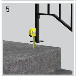
With the handrail setting plumb, measure the distance from the top step to the bottom of the upper post mount plate. This measurement is how much material you will need to remove from the bottom post.
