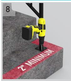
Make sure the posts are sitting a minimum of 2" from each side of the steps. Using a drill fitted with the included drill bit, drill through one of the holes on the post mount. Ensure you are drilling deep enough to accommodate the length of your fastener. For concrete, drill 3" deep, and for brick drill 6" deep.
