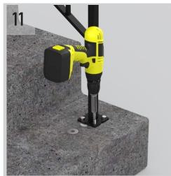
Select fasteners for your application, making sure that they are appropriate for the material you are drilling into, and secure the fastener into the hole that you have just drilled. Be sure to drill one hole and secure one fastener at a time. If the post is no longer level after fastening, place the included washers under the post mounts until a level reads plumb.
