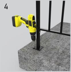
Using a drill fitted with the included drill bit, drill through one of the holes on the post mount. Ensure you are drilling deep enough to accommodate the length of your fastener. For concrete, drill 3" deep, and for brick drill 6" deep.
