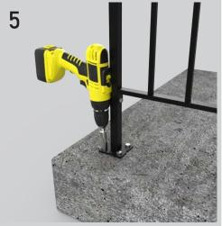
Select fasteners, appropriate for your platform material. Secure the fastener into the hole that you have just drilled. Be sure to drill one hole and secure one fastener at a time. If the post is no longer level after fastening, place the included washers under the post mounts until a level reads plumb.
