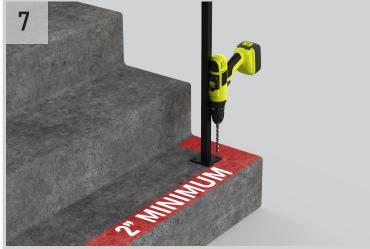
Make sure the posts are sitting a minimum of 2" from each side of the steps. Using a drill fitted with the included drill bit, drill through one of the holes on the post mount.
